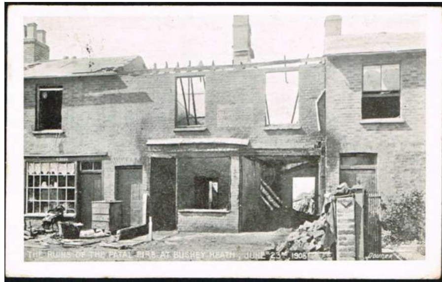
The aftermath of the fire
