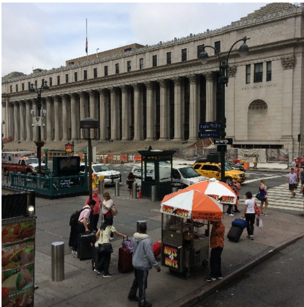
James A. Farley Post Office Building, with the inscription "Neither snow nor rain nor heat nor gloom of night stays these couriers from the swift completion of their appointed rounds."
