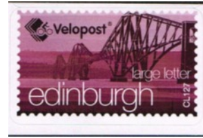
Edinburgh: Forth Bridge
