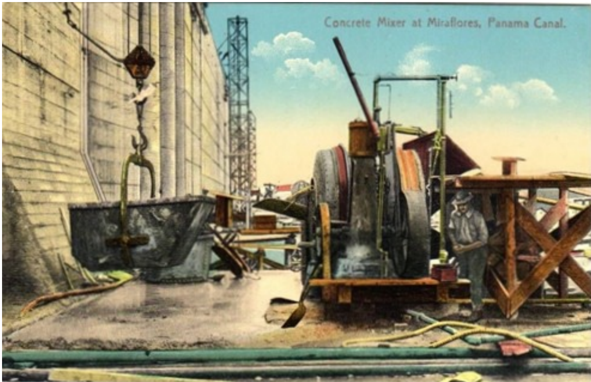
Concrete mixer at Milaflores Locks
