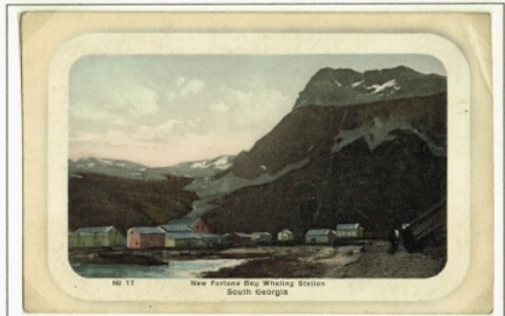
New Fortune Bay Whaling Station South Georgia was built by the Ocean Whaling Co., it closed at the end of 1920-21 season and the machinery moved to Stromness Bay.
